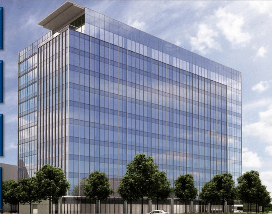
Enclave Place (Development – Expected Completion Summer 2015)
